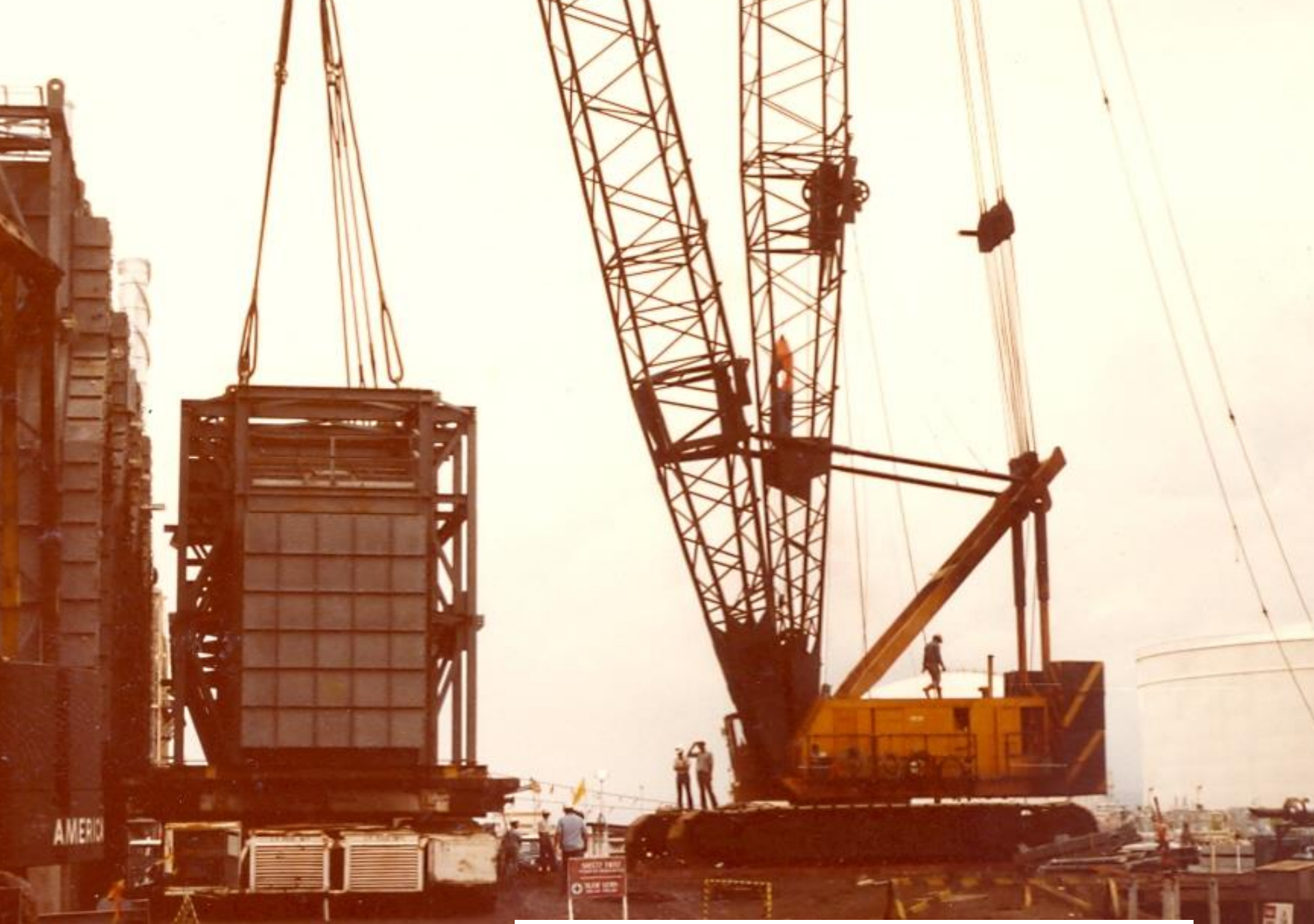
Heater section rigged to the hook
