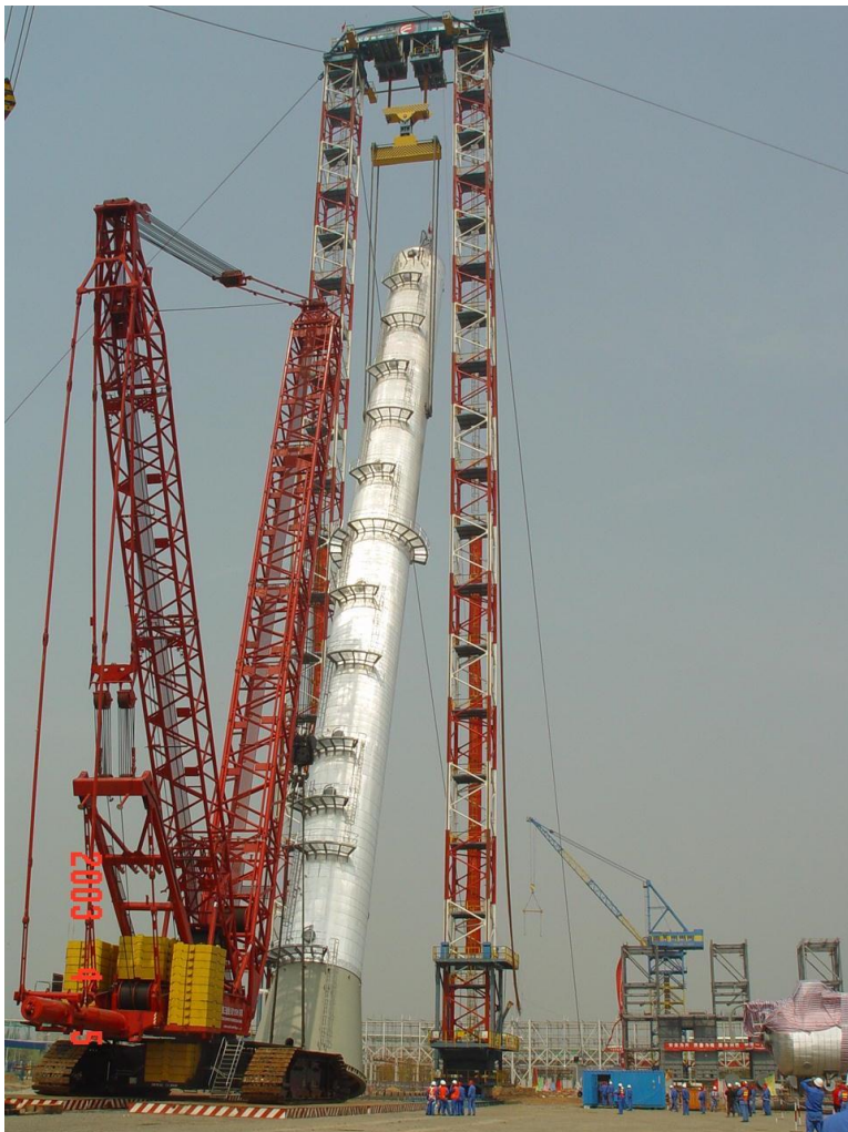
The next photo shows the dressed out rectifier being upended.
